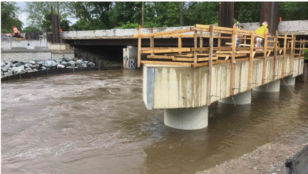
Photo 2: Pier construction for the new University Boulevard Bridge over the Northwest Branch Anacostia River
