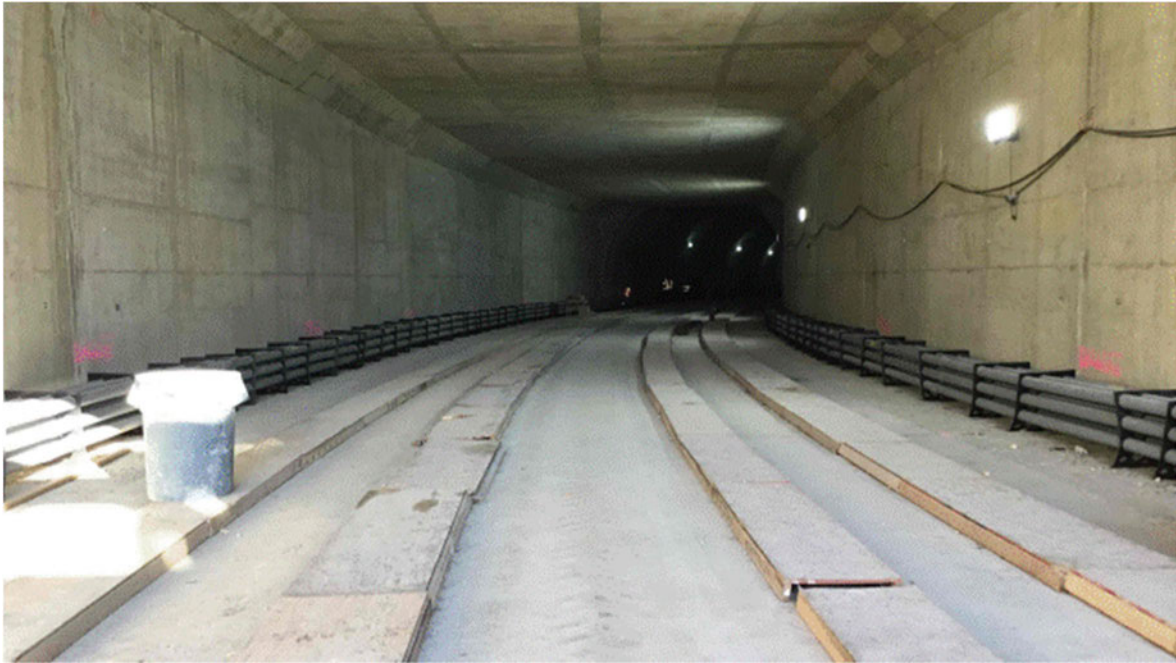
Photo 1: Communications Infrastructure Backbone ductbank (will be within the concrete maintenance/emergency walkway), East Cut and Cover section of Plymouth Tunnel.
