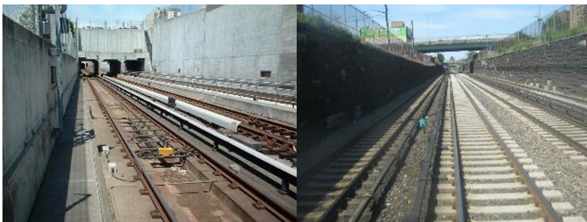
Figure C-22 U-wall construction
