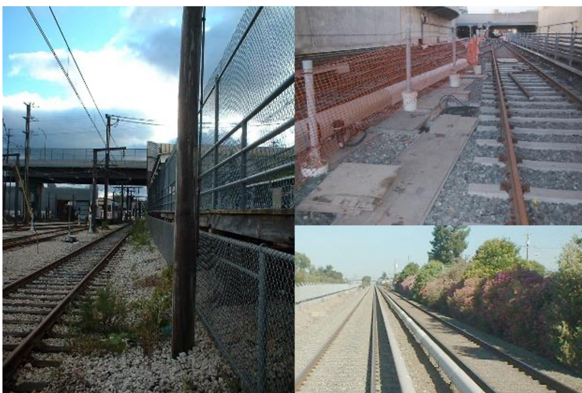
Figure C-14 Vegetation and fencing limiting PPOS
