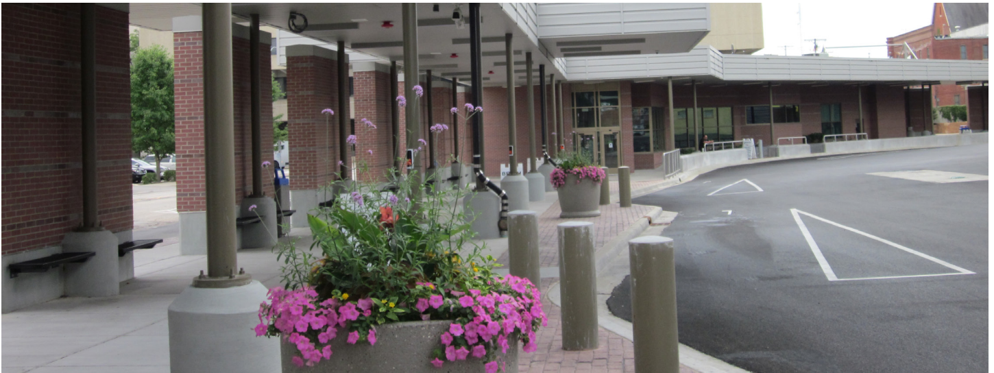
Figure 2-5. Image of Downtown Transfer Center
