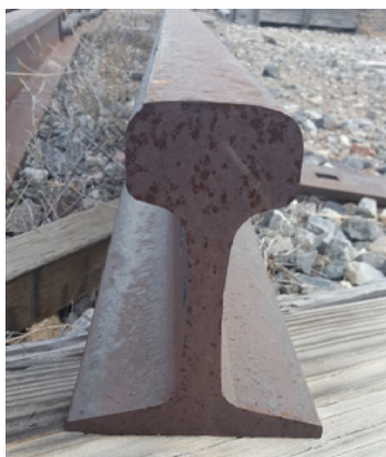
Figure 3-2 Cut section of rail
