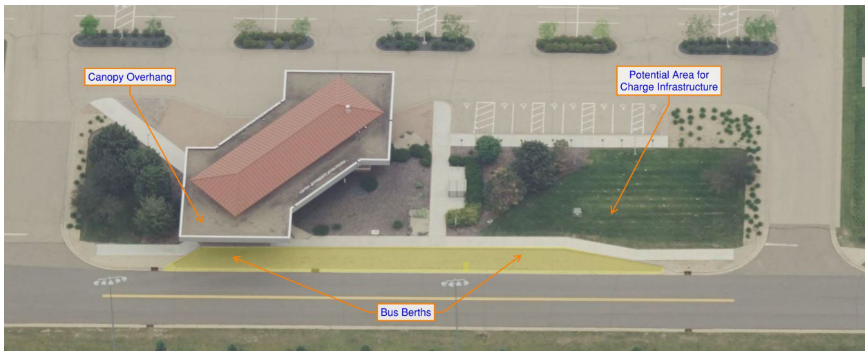
Figure 22: Aerial View of the 157th Street Station Passenger Berths
