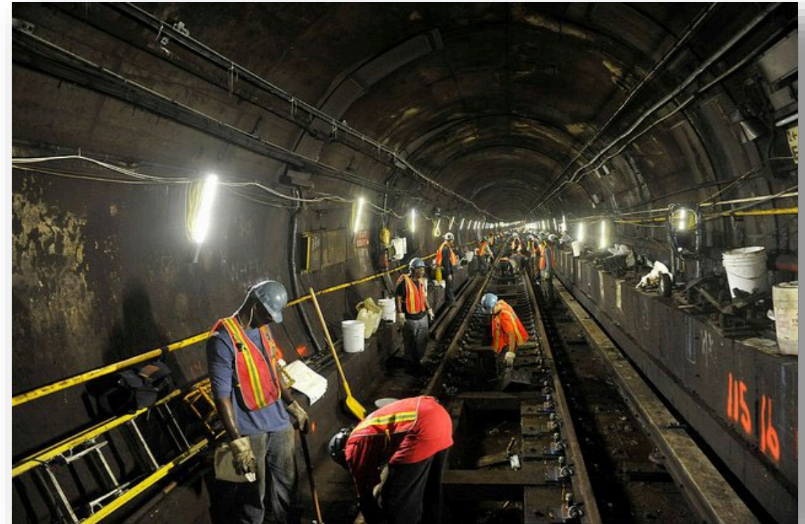
Hurricane Sandy repair work, MTA, New York, NY
