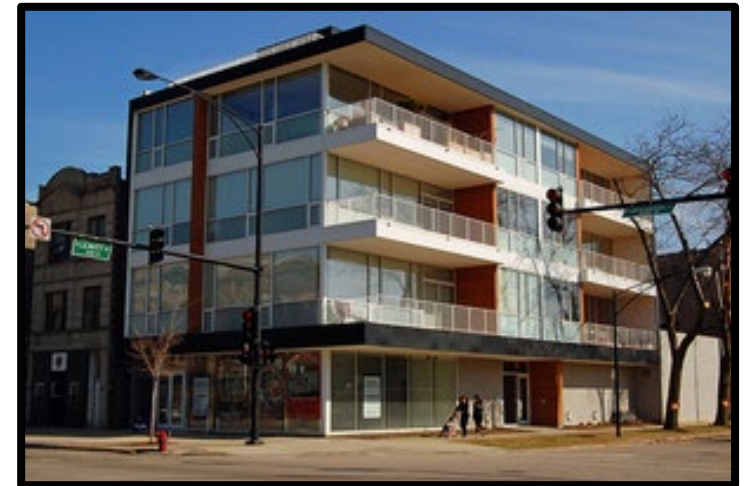
Mixed-use TOD development in Chicago, IL. Photo credit: Chicago Metropolitan Agency for Planning
