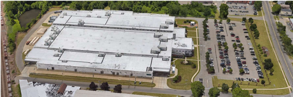
Figure 6.2: CTtransit New Haven main facility
