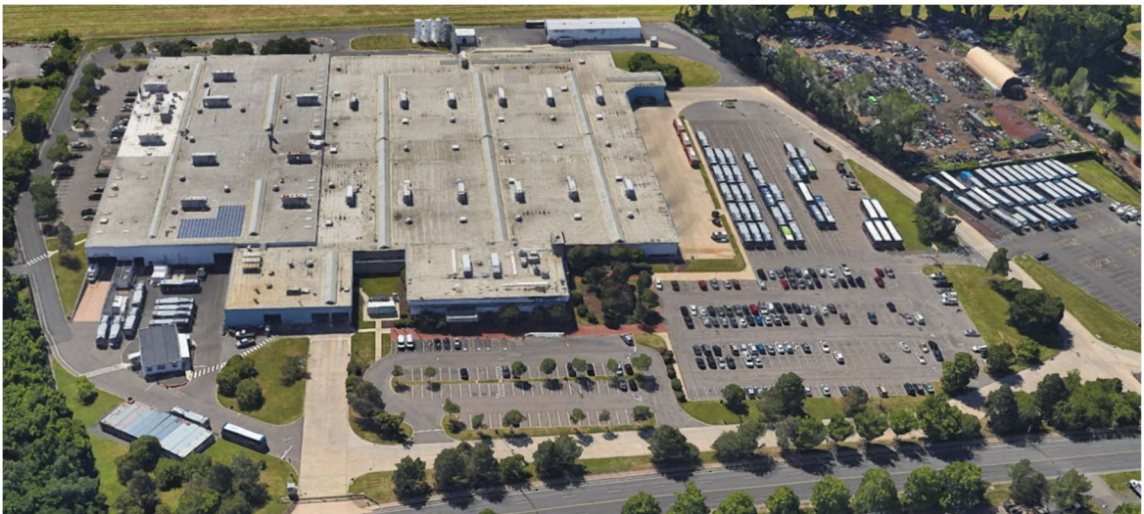
Figure 6.1: CTtransit Hartford main facility
