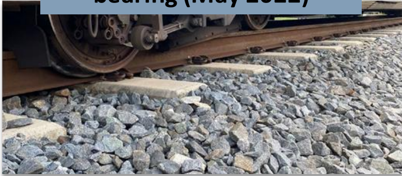
CATS derailment and failed bearing (May 2022)
