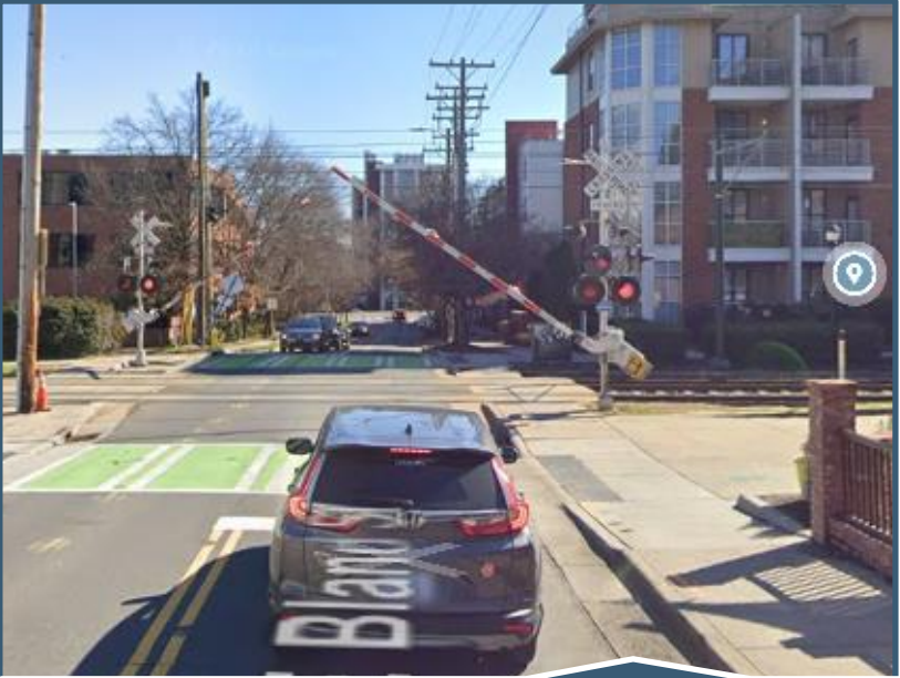
Rail Crossing Gates
