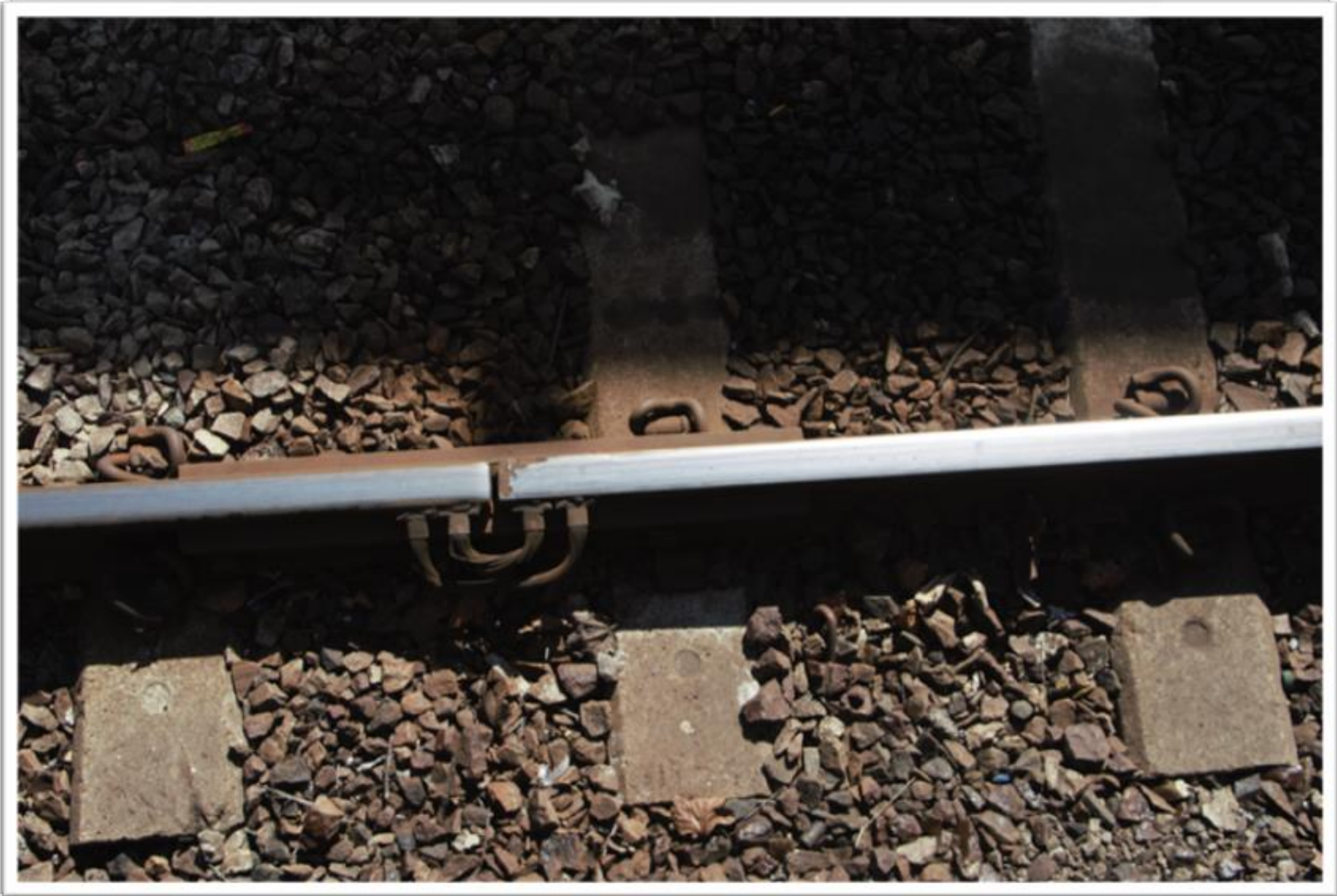
Photo depicting rail end batter
