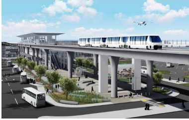
Los Angeles World Airports Automated People Mover (currently under construction)
