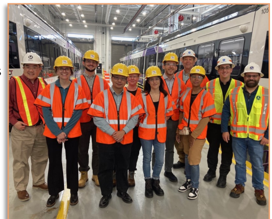
TSO's Office of System Safety visits Maryland's Purple Line construction in November 2024.
