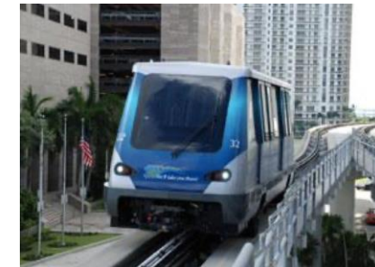
Monorail/Automated Guideway (MG)
