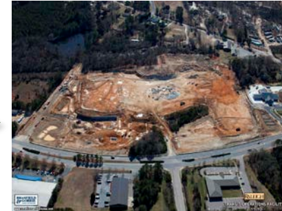
Notice to Proceed Site Construction
