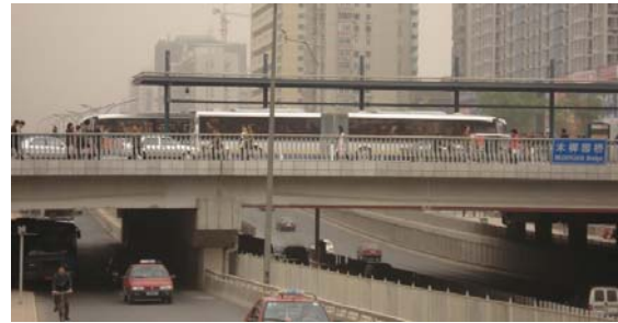
Beijing BRT Line 1 Station at Arterial Overpass
