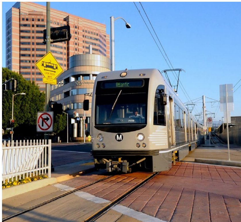
Figure 4A-6 Gold Line, Los Angeles
