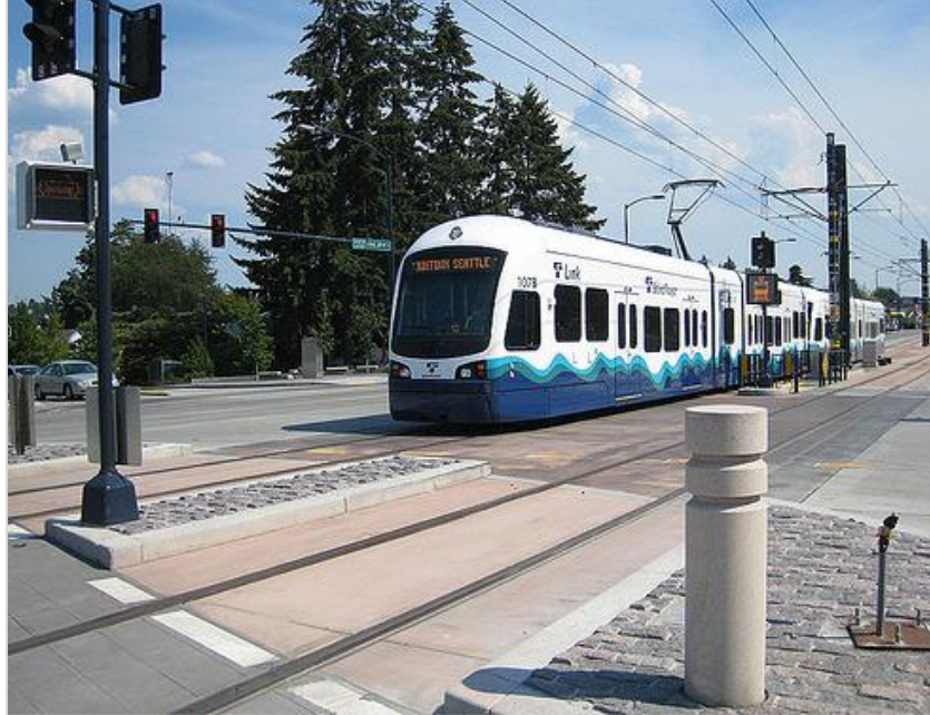
Figure 3. Embedded Track used by Link Light Rail. 4
