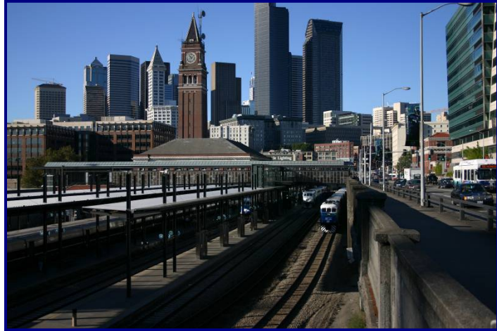
Figure 10: View of Seattle Skyline over King Street Station
