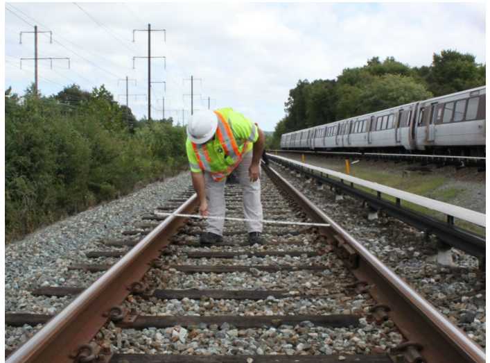
FTA Lead Safety Investigator Troy Lloyd checks track gauge along the WMATA Metrorail track.
