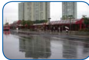
Ottawa Transitway Intermodal Station
