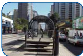
On-Street Island Platform in Curitiba—RIT
