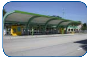
Extended bus platform on Miami-Dade Transitway
