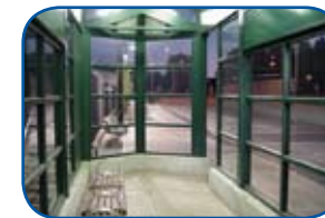
West Busway facility in Pittsburgh
