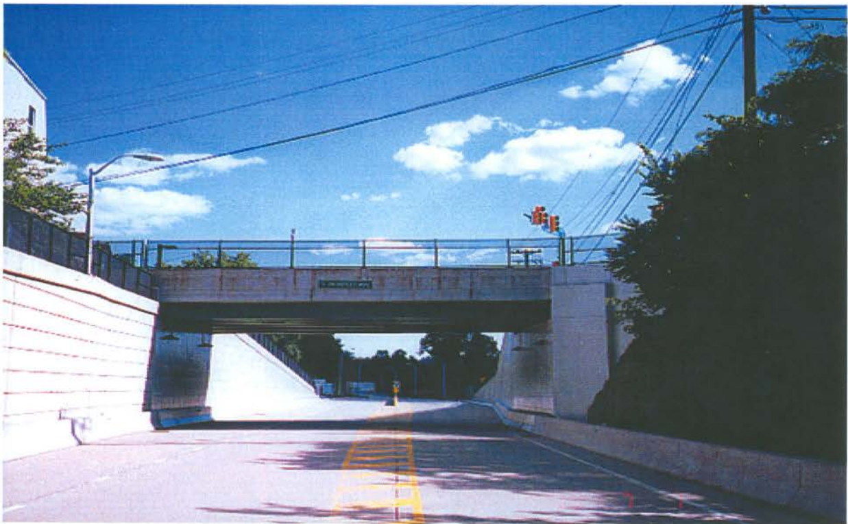
East Prospect Bridge – After
