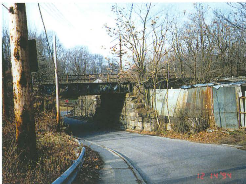
Railroad Bridge At Morrance Road Prior to West Busway Construction
