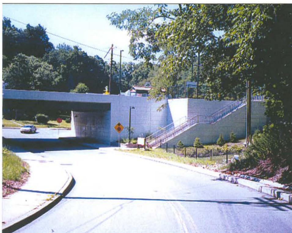
West Busway Bridge at Morange Road
