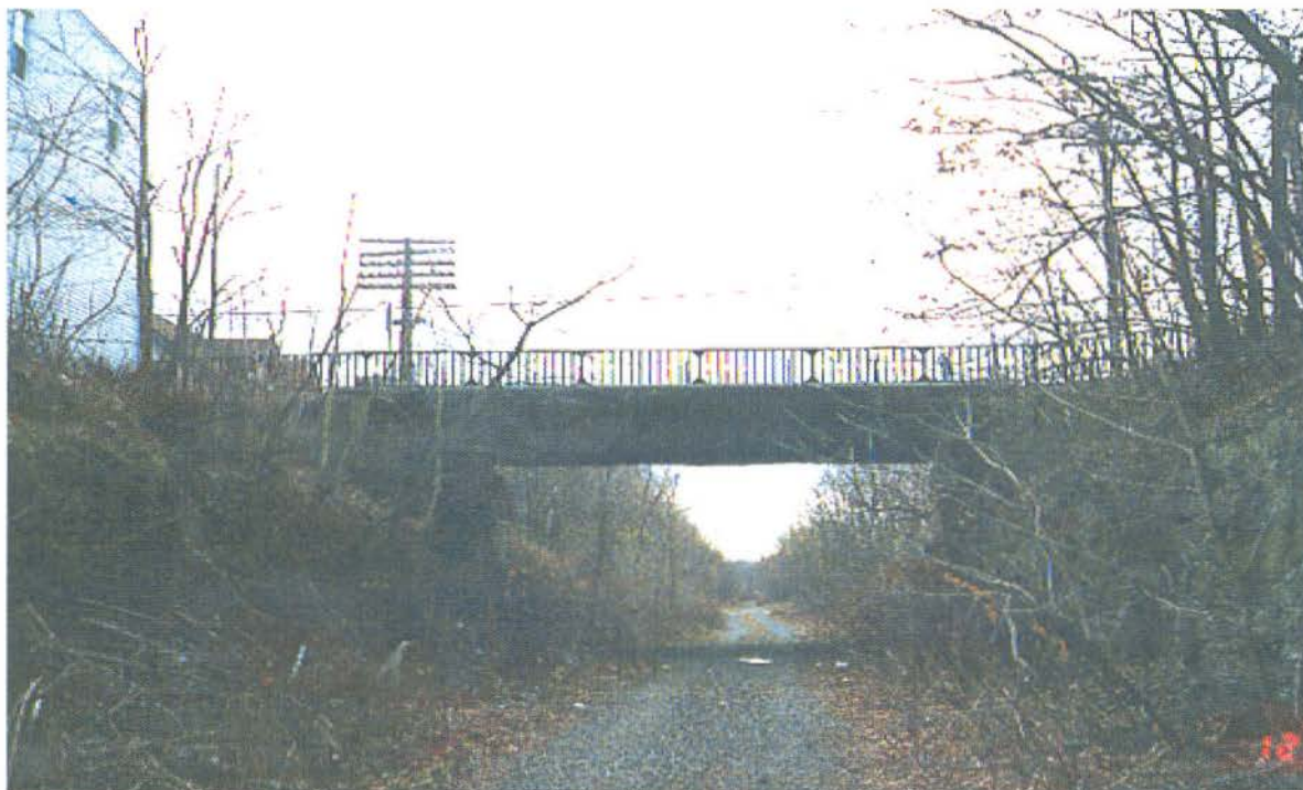
East Prospect Bridge – Before
