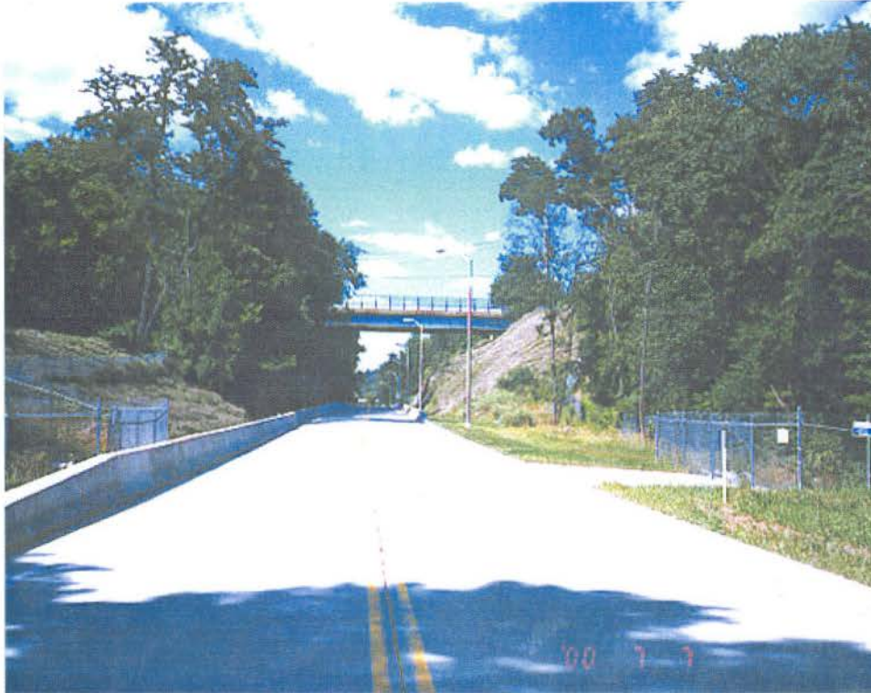
West Busway at Crennell Avenue
