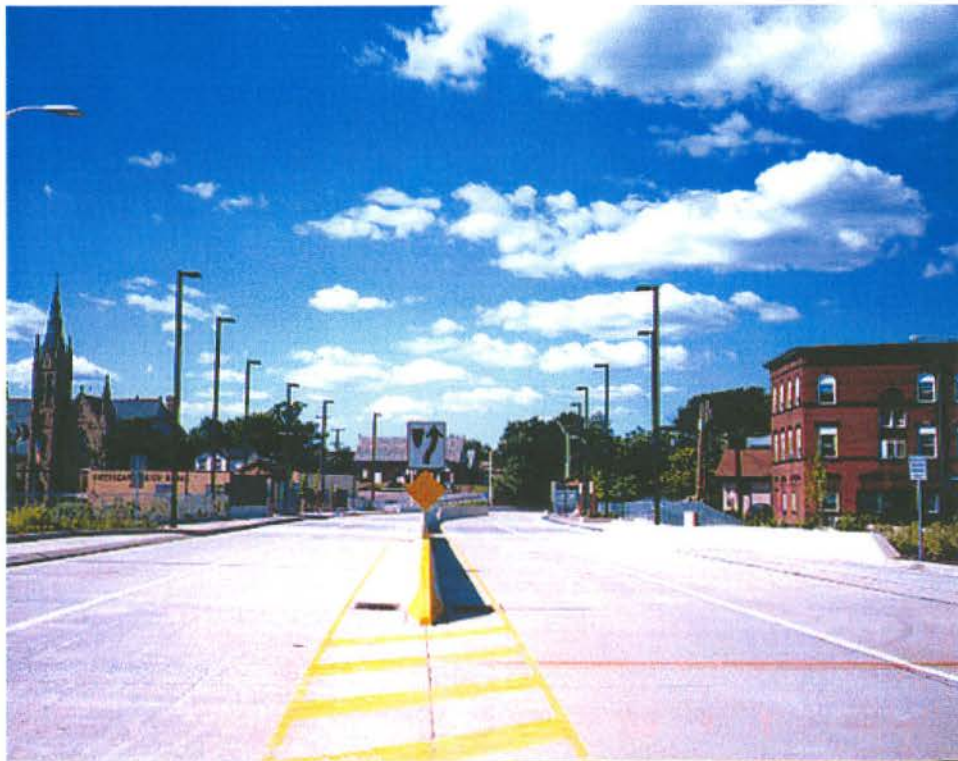
West Busway Crafton Station
