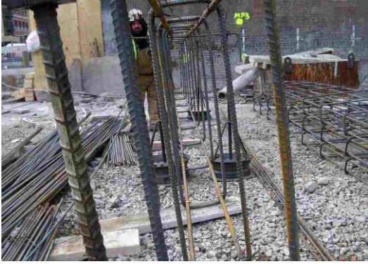
C2A – Installation of Secant Pile Guide Wall at Ancillary 2 -- W Corner of 97 th St. and 2 nd Ave.
