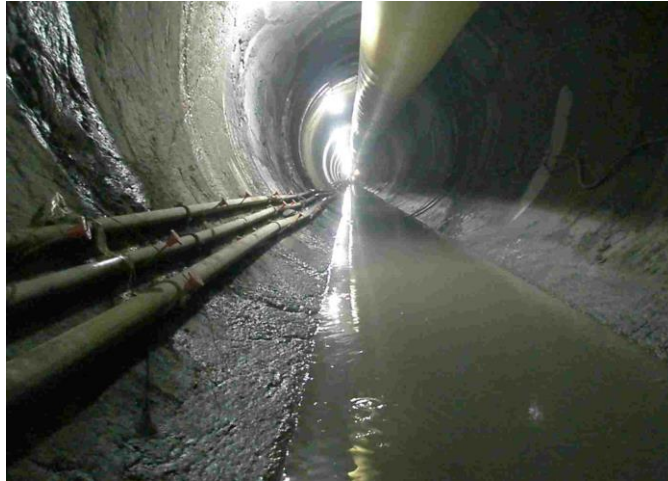
C1 – West Tunnel – Currently 5,978 linear feet
