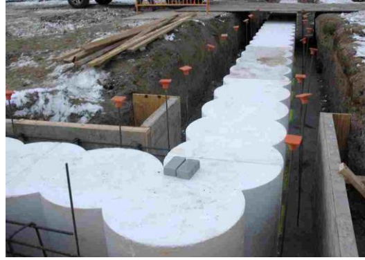
C2A – Installation of Secant Pile Guide Wall at Ancillary 2 -- W Corner of 97 th St. and 2 nd Ave.
