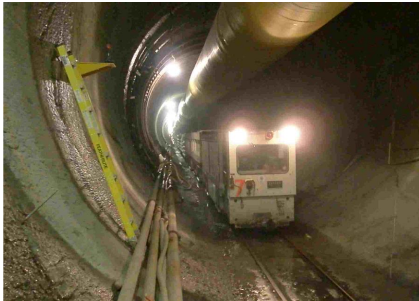
C1 – Muck Train Removing Rock from West Tunnel
