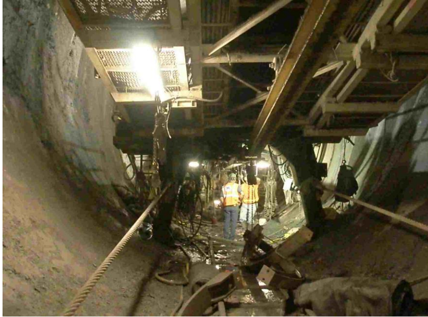
C1 – Tunnel Boring Machine in West Tunnel
