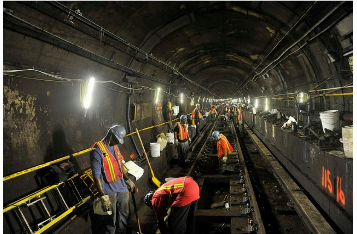
Hurricane Sandy repair work, New York, NY
