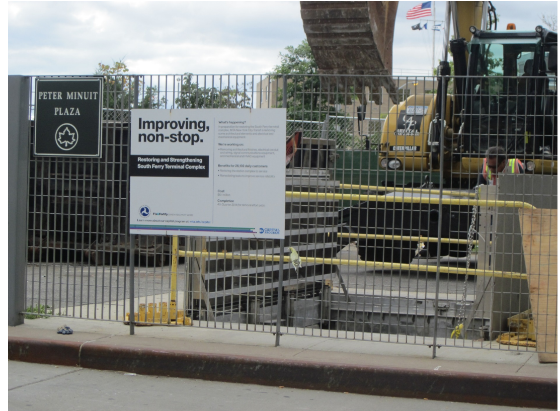
South Ferry Station resilience project, New York, NY - 2014
