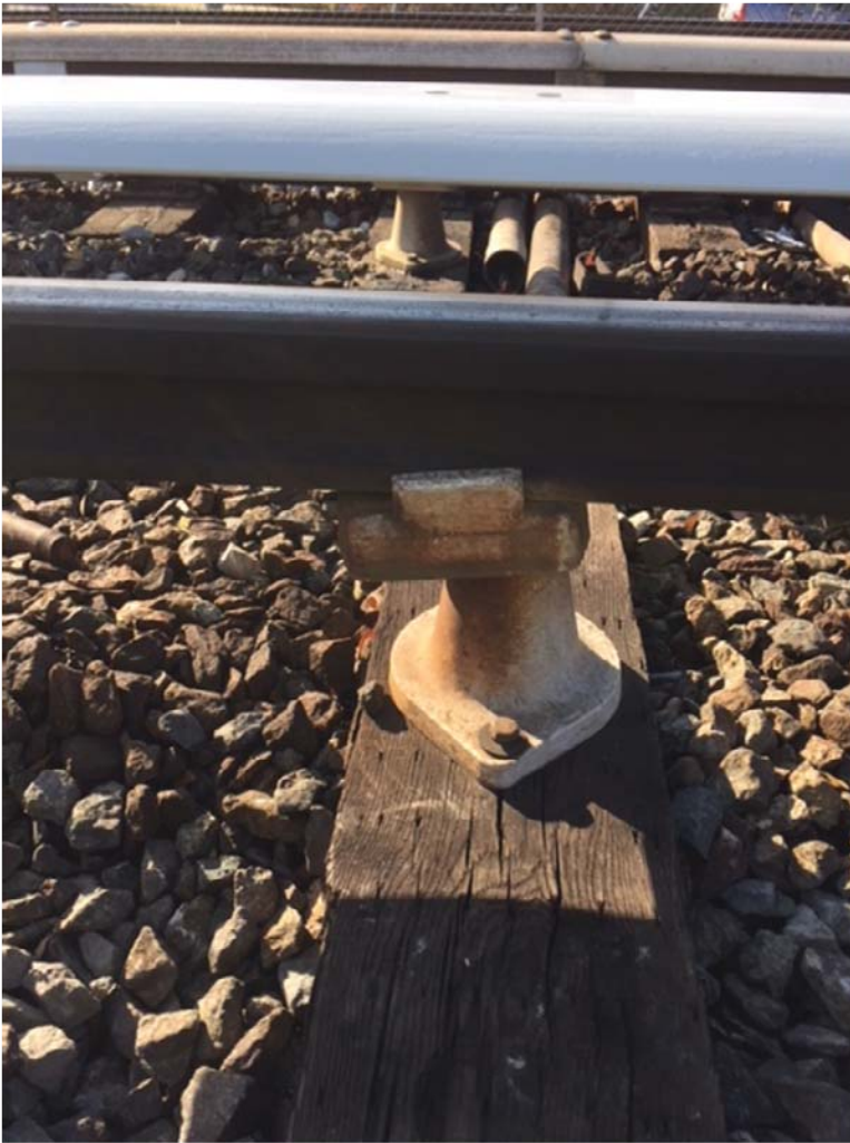
Figure 1: Defective insulator at B1 349+90.
