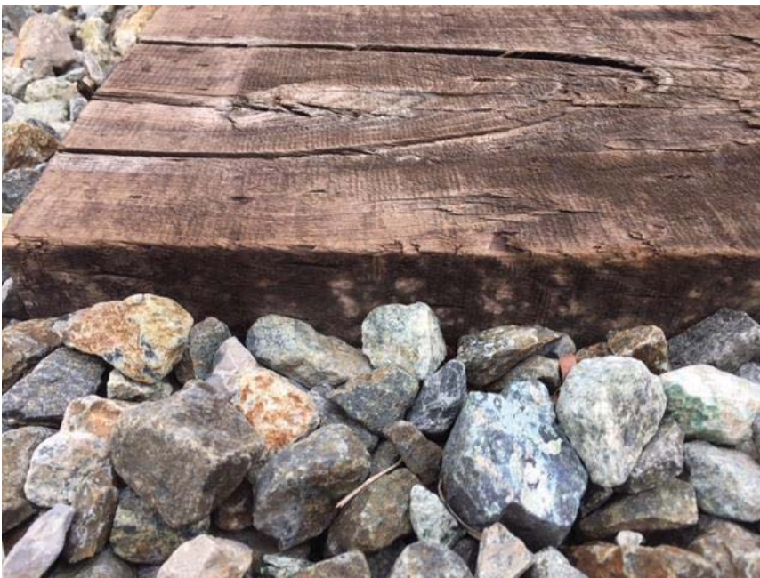
Figure 4: Ballast marks on the side of ties demonstrating deflection between Brookland (B05) and Fort Totten (B06).
