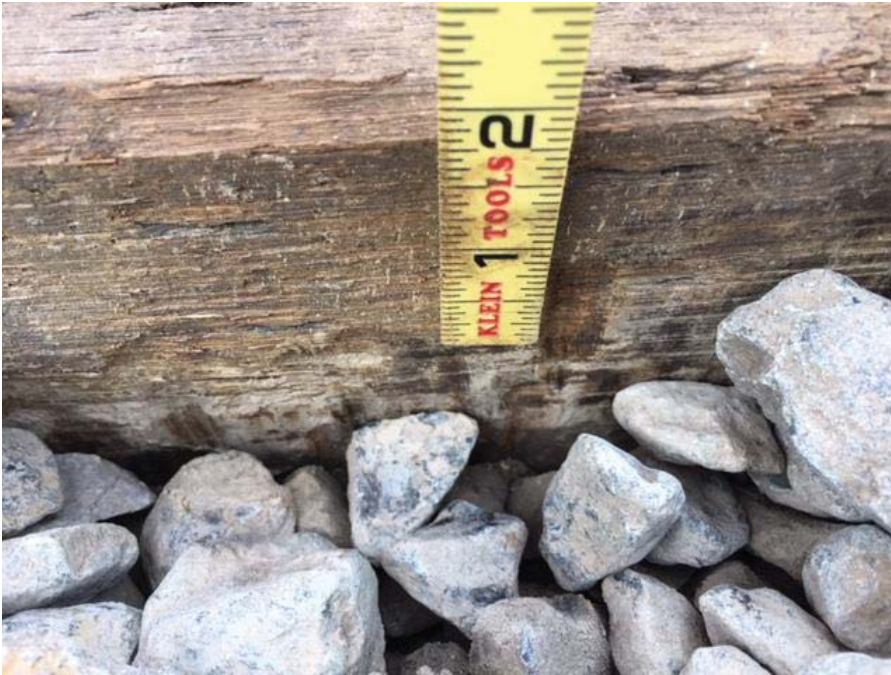
Figure 3: Ballast marks on the side of tie demonstrating vertical deflection under load at D2 294+80.
