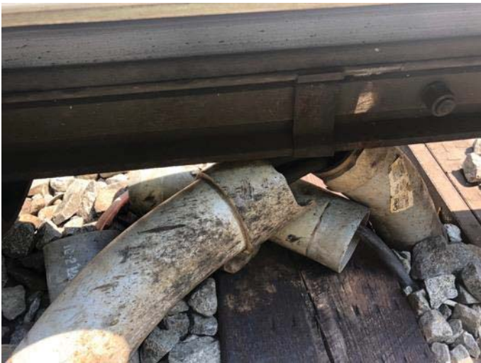
Figure 2: Cables and conduit underneath third rail at F1 408+50.
