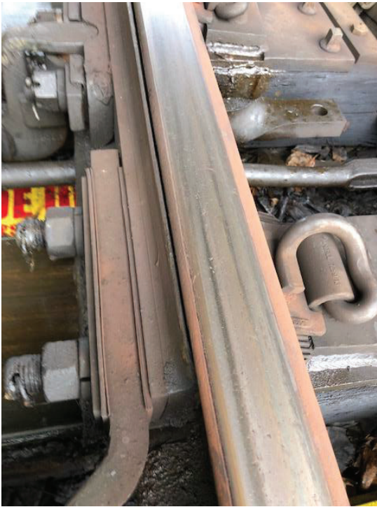
Figure 1: A1 937+10 at the 3A switch, right side point gapped 3/16-inches.
