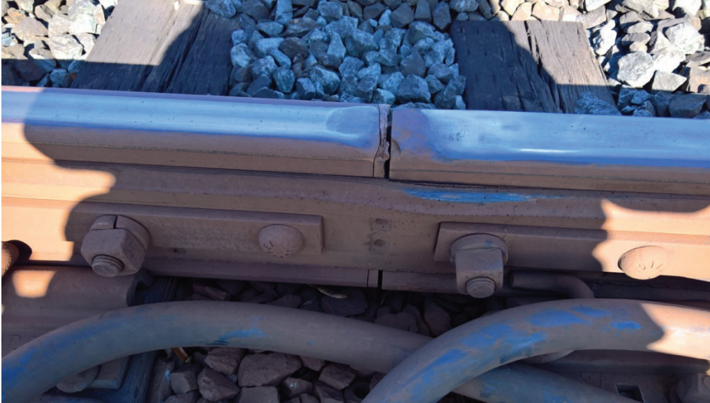
Figure 1: Insulated Joint at CM K1 772+20.
