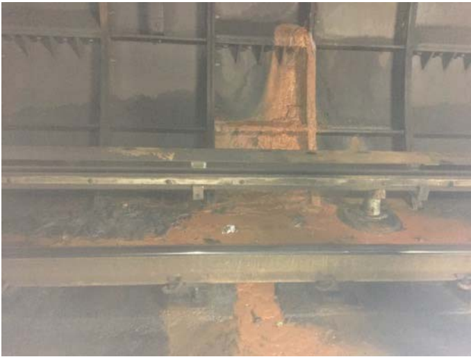
FIGURE 1 – F1 081+00 – STANDING WATER SURROUNDING 3 RD RAIL INSULATORS.
