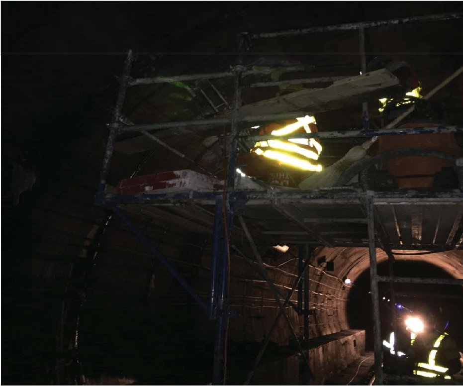
Figure 1: Crews on mobile scaffolding drilling 3/4-inch holes through the tunnel liner into the bedrock above the lining at the source of the water.
