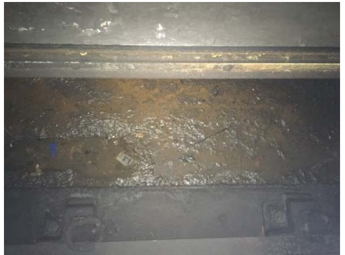
FIGURE 2 – F1 144+00 – STANDING WATER SURROUNDING POWER FEEDER CABLE CONDUIT STUB-UPS.
