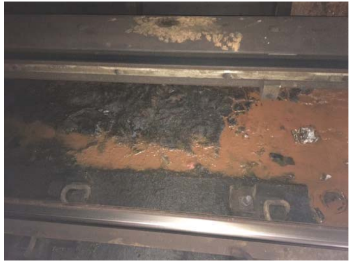
FIGURE 1 – F1 081+00 – STANDING WATER SURROUNDING 3 RD RAIL INSULATORS.
