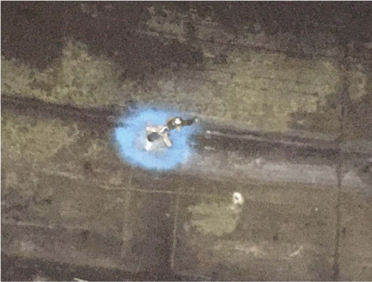
Figure 5: Cylinder/valve injection device placed into the hole prepared for solution injection.
