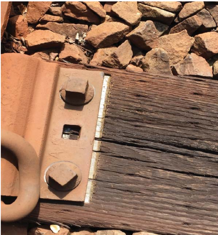
Figure 2: Field side plate movement at F2 401+00.
