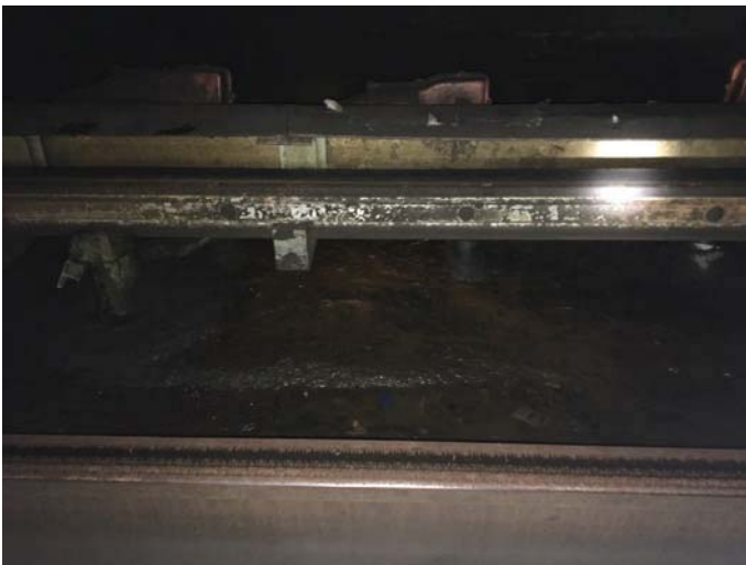
FIGURE 2 – F1 144+00 – STANDING WATER SURROUNDING POWER FEEDER CABLE CONDUIT STUB-UPS.
