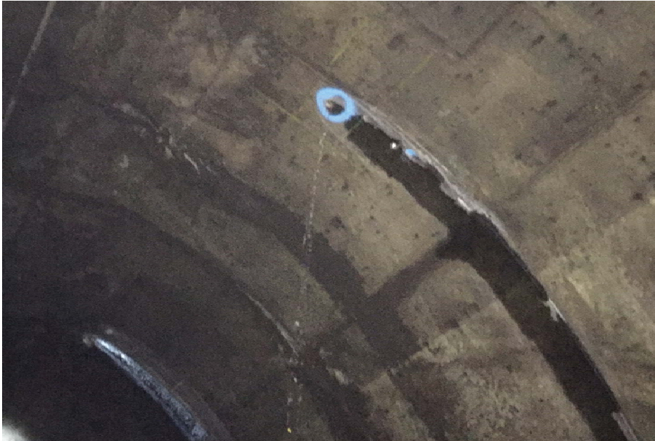
Figure 2: After holes are bored, water was released from the entering source.
