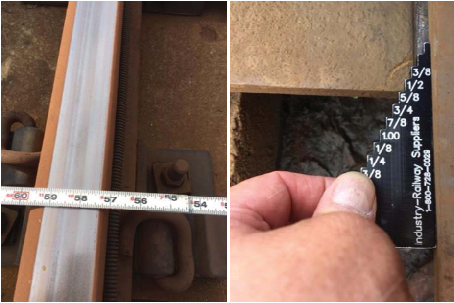
Figures 4 and 5: 1B switch 57-1/4 static gauge with 3/8-inch dynamic movement (57-5/8) at C2 622+00.
