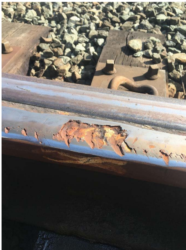
Figures 3 and 4: Spalling and rail head crack on the straight closure rail of the 11A switch at B2 116+20.
