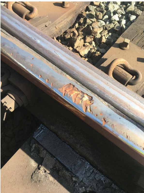
Figures 3 and 4: Spalling and rail head crack on the straight closure rail of the 11A switch at B2 116+20.
