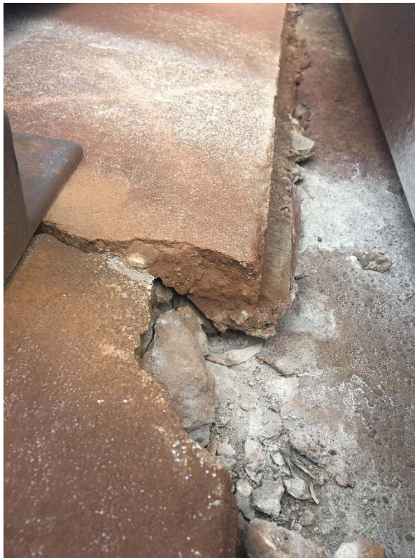
Figures 1 and 2: Defective fasteners and deteriorating grout pad between B2 144+00 and 145+00.
