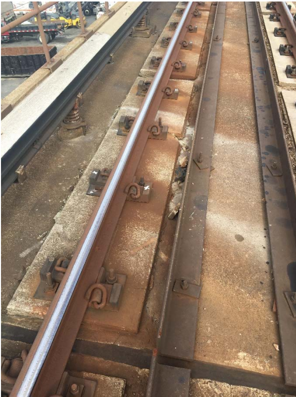
Figures 1 and 2: Defective fasteners and deteriorating grout pad between B2 144+00 and 145+00.
